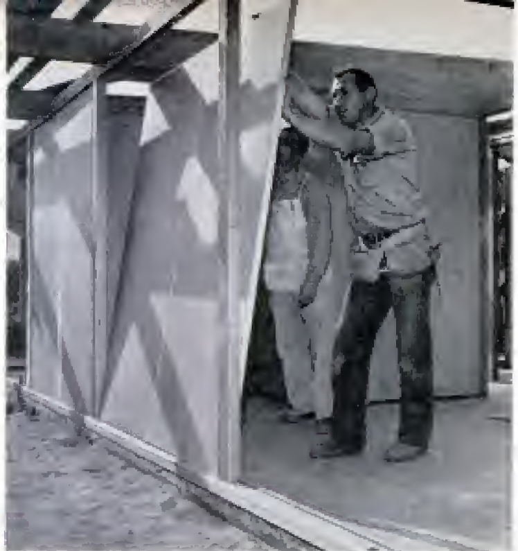
Carpenters raise pair of exterior wall panels into place. Interior space saved by thin walls amounts to 150 square feet
